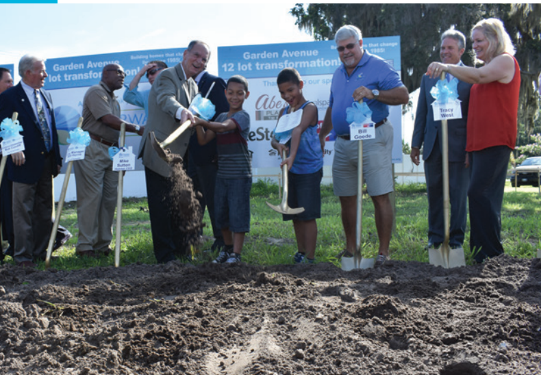
Garden Avenue Groundbreaking of 12 lots in the North Garden Avenue Marina District of Clearwater, FL
